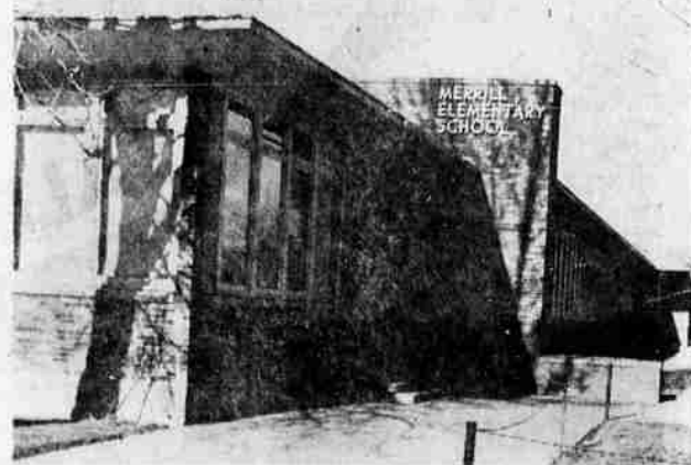
New Merrill elementary school, thoroughly modern, and a credit to any community!
