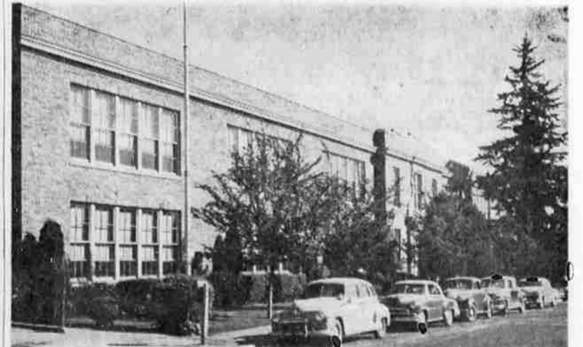
FREMONT School houses both the eighth grade and primary classes. It was constructed in 1925 to replace the old Central School. It was named for General John C. Fremont, famous explorer, who visited the vicinity of Klamath Falls in 1853 and again in 1856 on exploring expeditions. The school handles 45 in the primary and 335 eighth graders.
