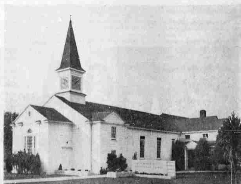
RE-EVALUATION of the present room structure of Peace Memorial Presbyterian Church, South Sixth Street, will eventually lead to remodeling of the present structure. A wing was added some time ago. Work projects to provide for extra space for classrooms continue as needed. The church board recently purchased a large parking lot west of the original property to be developed during the coming year as funds are available. The white church is one of the most attractive in the city.
