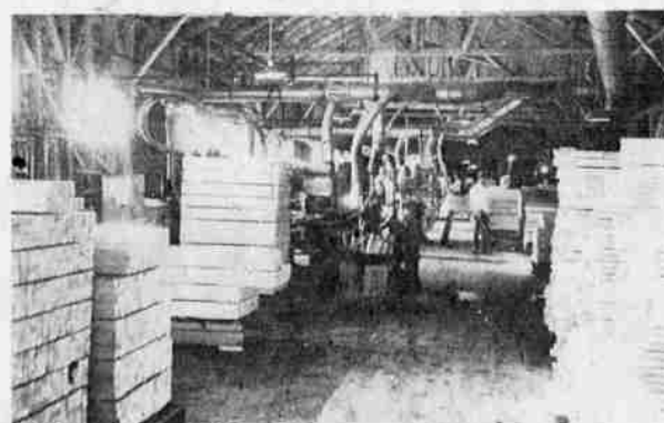
Part of general machine area showing principal machines used in manufacturing of frames and windows.
