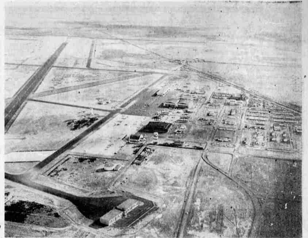
THIS AERIAL VIEW of Kingsley Field shows the layout of one of the Air Defense Command's newest bases. The flight line and F101-B "Voodoos" are lined up in the middle of the picture. The FAA control tower is at the left of center and the main north-south runway is at the extreme left. The alert hangar, where air and ground crews stand 24-hour alert, is at the bottom of the picture. Kingsley Field is an important factor in the continued progress of the Klamath Basin as it contributes nearly $10 million a year to the economy.
