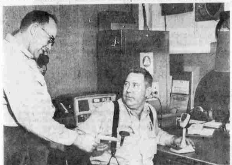
FROM THIS STATION at the Suburban Fire Department headquarters dozens of volunteer firemen may be alerted instantly. This office also serves as a civil defense warning point. The men are Roger Wilkinson, a driver, standing, and Joe Sullivan, engineer.
