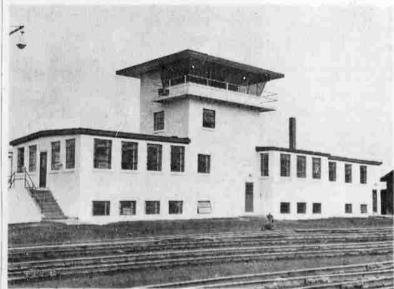
A NEW YARD OFFICE for Great Northern was unveiled in 1958. The building was constructed at a cost of $140,000 and houses radio communication equipment designed to facilitate the movement of rail traffic in and out of the area.
