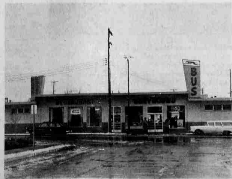
NEW FACILITIES for bus travelers were provided with this new terminal which was dedicated in 1958. The terminal cost an approximate $125,000 and features the most modern facilities including a Greyhound Post restaurant. The building provides canopied dispatch service space for seven buses at the rear of the structure.
