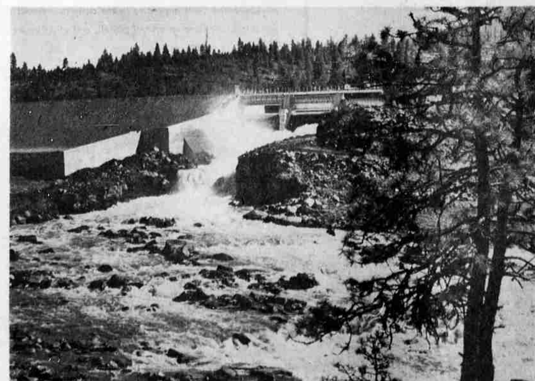
THE HARNESSING of the potential power of the Klamath River received a giant boost when the Big Bend project was completed and dedicated on Oct. 2, 1958. This plant will generate 80,000 kw. The view shown here was taken behind the giant earth fill dam across the Klamath River. Water from this point flows through a concrete flume and drops 819 feet through twin flumes to the powerhouse in the canyon. The dam at this point is 652 feet wide. Work is already underway on the Iron Gate Dam in Northern California.
