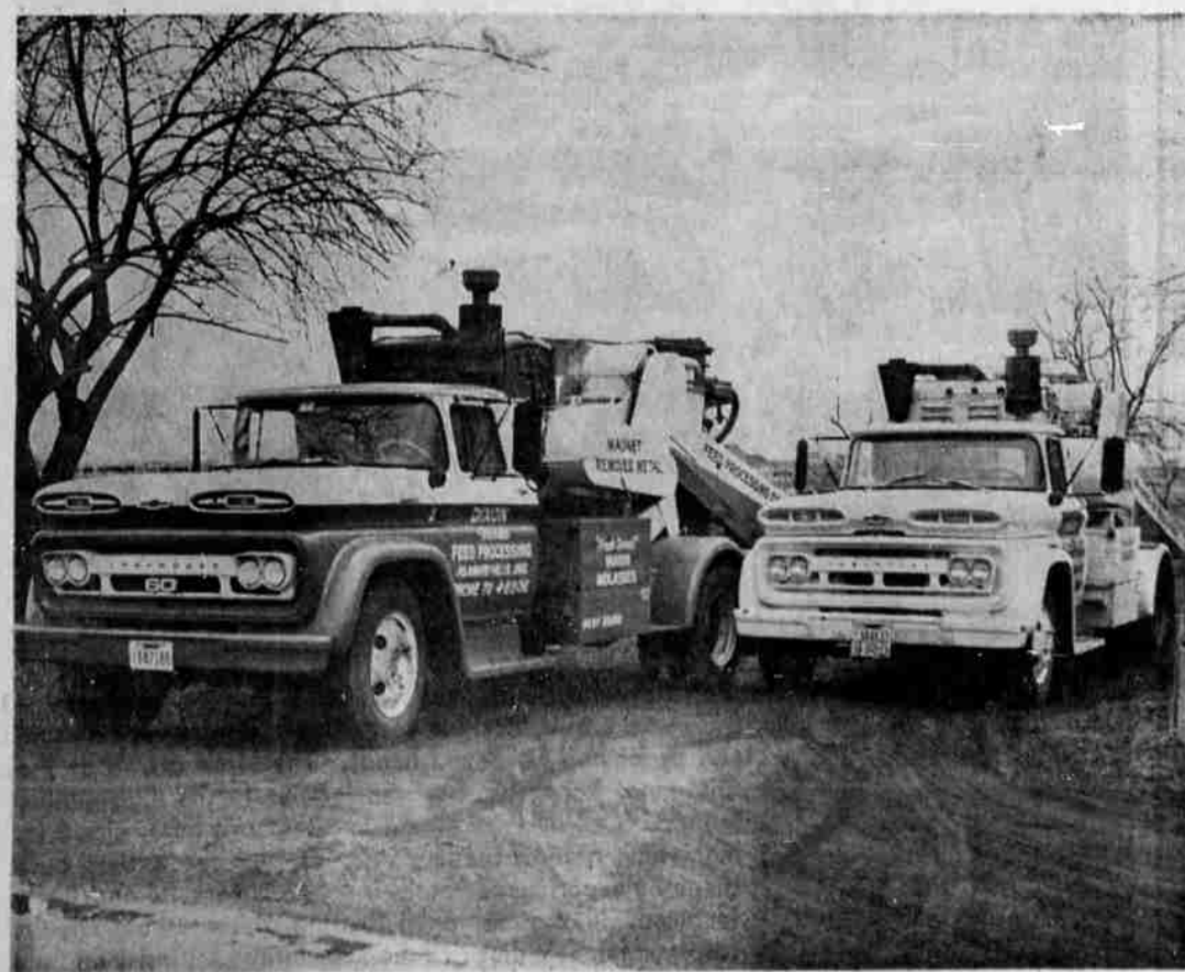
The two big Daffin Mobile Feed U-Nits follow a regular route system throughout most of the Klamath Basin offering complete on-the-farm feed processing service. All grain can be handled through the air loading and unloading system. Baled hay, of course, must be hand fed.
