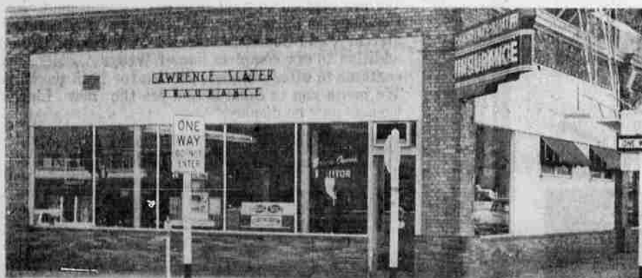
An outside view of our modern offices located at 7th and Pine Streets.
