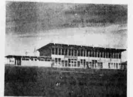
Fremont Glass & Millwork installed all the glasswork in Klamath's New Airport Terminal Building.
