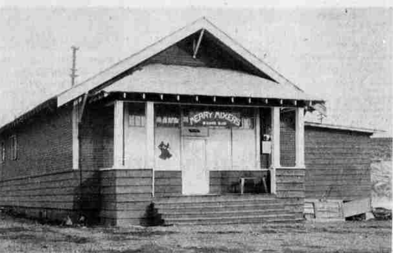
HOME OF MUSIC, fun and frolic is this headquarters for the Merry Mixers Square Dance Club. It was a former store and had been unoccupied for a number of years prior to being purchased and completely remodeled by the club members into their own hall.
