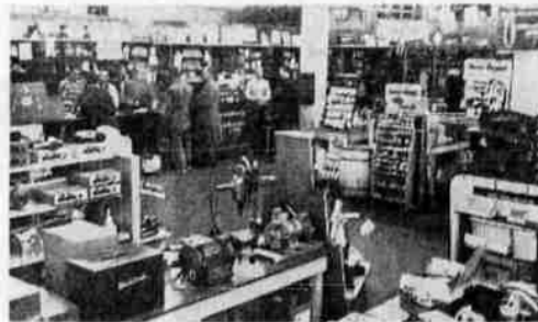
An inside view of the main stock room in the Klamath Falls store.
