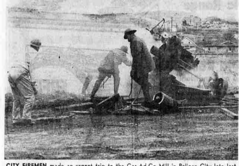
CITY FIREMEN made an urgent trip to the Car-Ad-Co Mill in Pelican City late last week to find this unused piece of machinery afire in the yard. Damage was confined to the machine.
