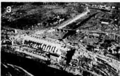
A new power project solves both problems.
