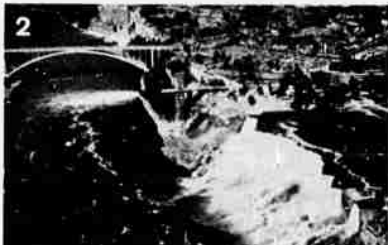
Other erosion defaced the Falls itself.
