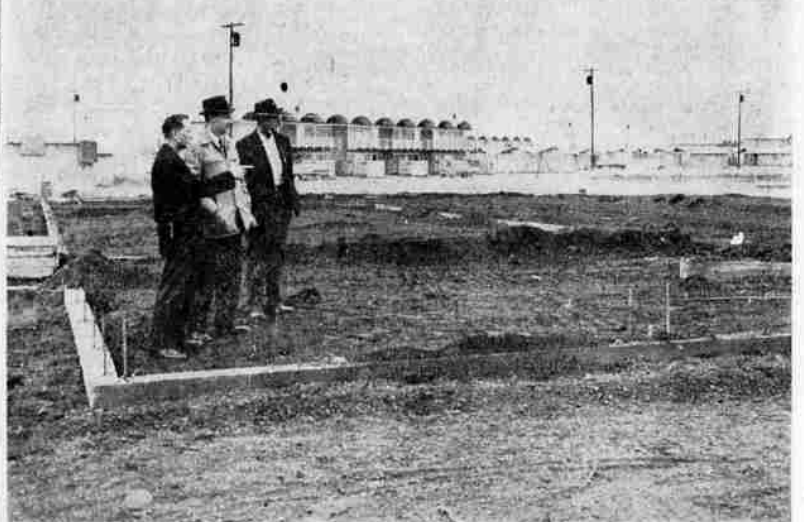
THE FOUNDATION for the new restaurant, about 6,000 square feet of floor space, has already been poured and construction underway on this site, being examined by, left to right, Arthur Rickbeil, Don Sloan and George Brosthouse. Completion date has been set for June 1.
