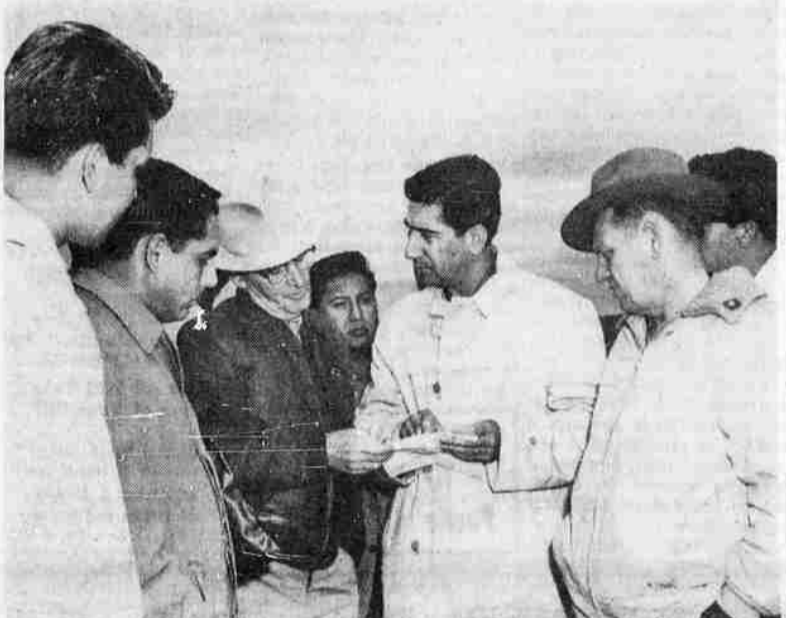
OFFICIALS OF THREE pipe-laying companies in two countries are shown here discussing the itinerary of a 16-man Mexican group here to observe American pipe-laying methods. Bill Blake, third from left, resident engineer for Bechtel Corporation, discusses an itinerary with Octavio Ruiz, third from right, superintendent of construction for the Mexican government petroleum company, Pemex Petroleos Mexicanos. Joe Eakin, second from right, office manager for H. C. Price Co., looks on with other Mexican engineers.
