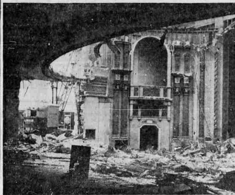
LOOKING LIKE the bombed out interior of a cathedral is this inside view of the Pelican theater as it continued to disintegrate into rubble in the smoothly planned demolition to clear the site for a parking lot. The reinforced concrete slows the rate of destruction, but everything is progressing as planned on this community landmark. Photographer Don Kettler got this unusual view late last week.
