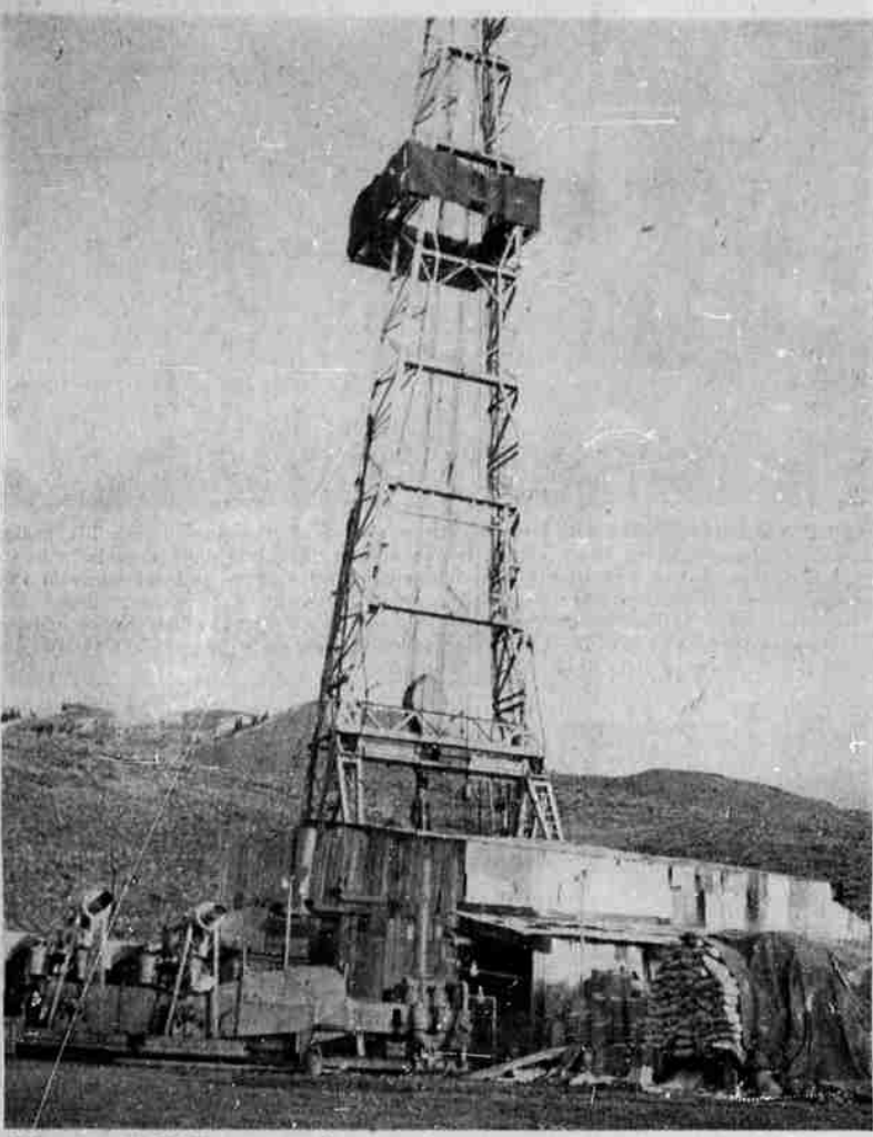
THIS OIL DERRICK rises 156 feet into the sky about four miles south of Lakeview. Drilling operations continue and have reached a depth of 7,850 feet. The Sun Drilling Company is conducting the drilling on a contract basis for the Humble Oil Company.
