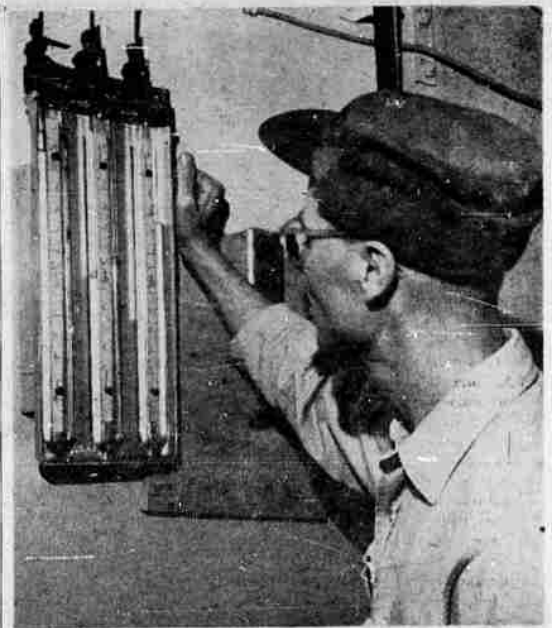
CHECKING the accumulation of methane gas in the dome of the digester at the city sewage disposal plant is Bill Swanson. He keeps careful tabs on the gauge indicators of gas produced in the digesters. Paul Barnes is superintendent of the city sewage disposal plant.
