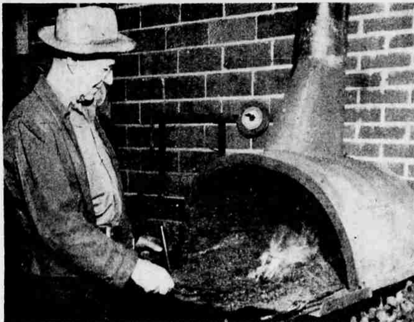
THE DAY wouldn't be complete for George Earnest if he didn't drop in at the GE Forge and Tool Works to have a look around. The business is now owned by Adam Eckerich who plans to expand to meet demand. Earnest, the proud blacksmith, is shown heating up some iron in the shop.
