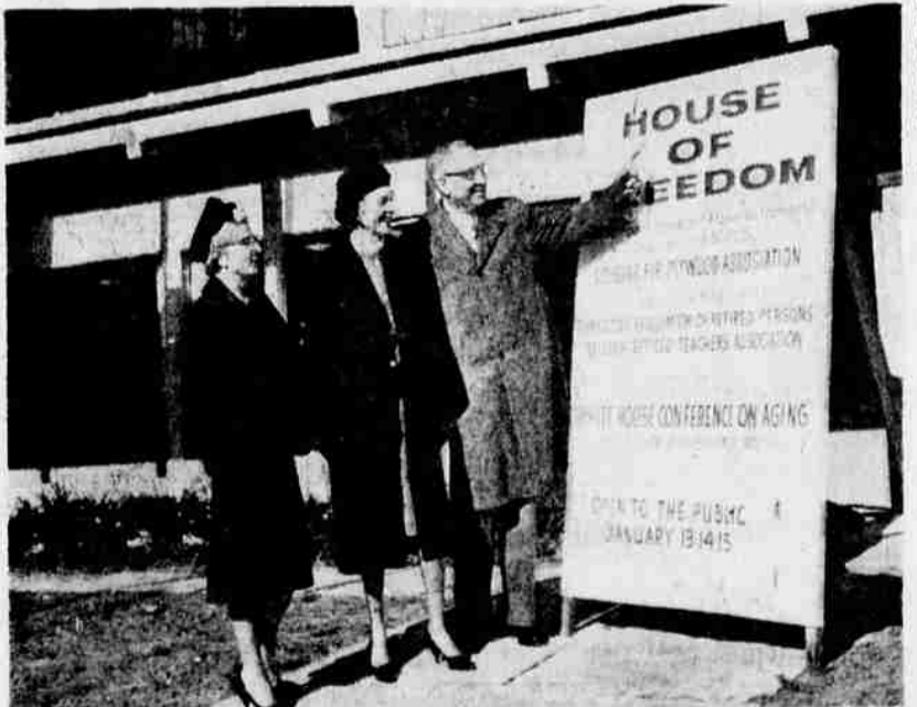
A COMFORTABLE $9,000 HOME, designed for Americans over 60 years of age, was a special Washington, D. C., attraction during the recent White House Conference on Aging. The two-bedroom home shown here was constructed from Western lumber. It uses three times the usual amount of plywood. Sen. Maurine Neuberger, center, visited the demonstration house recently, along with Mrs. Clifford Zollinger, left, Portland, member of the Oregon State Council on Aging, and Eli McConkey of Astoria. Sen. Neuberger expressed hope that construction of such homes would help Oregon's plywood industry.
