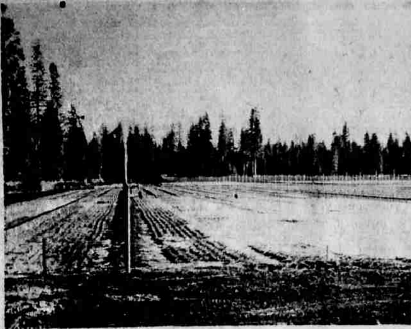
THE FOREST SERVICE TREE FARM covering 52 acres near McCloud is receiving new facilities, including two offices, a laboratory, a cold room and seed handling room to facilitate annual production of 10 million two-year-old seedlings. — Photo by Ray Kite
