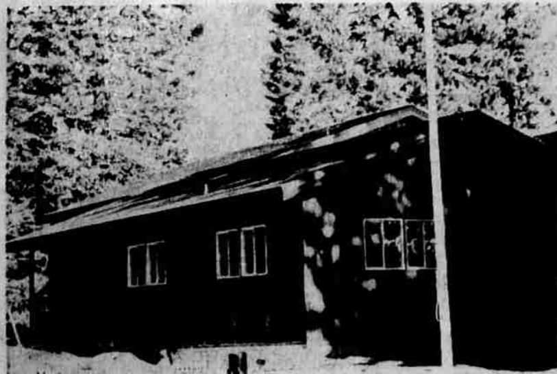
A CLOSEUP VIEW of a new redwood building that is among new facilities built at Mt. Shasta Tree Nursery east of McCloud on Highway 89. The problem of seed storage needed for increased production was solved with addition of a new cold room. Seeds may be stored indefinitely, said Karl Lanquist, superintendent. — Photo by Ray Kite
