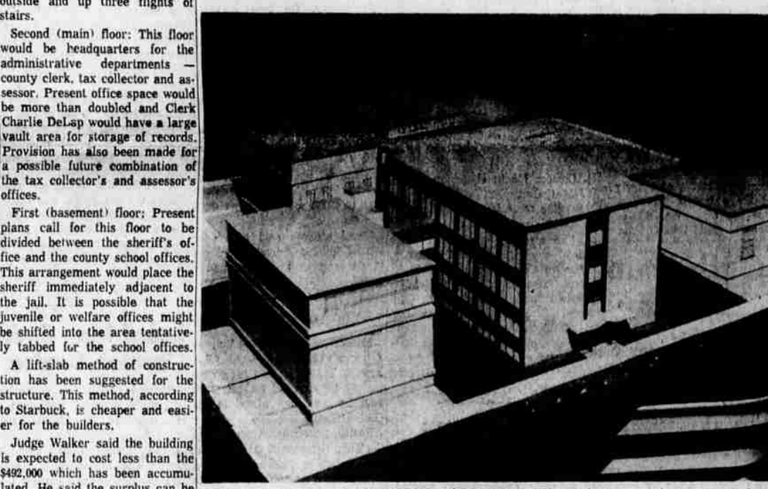
THE FOUR-STORY COURTHOUSE ADDITION is shown here in scale in a view from the rear of the courthouse. The new addition, to be built in what is now the parking lot, will be 118 feet long and 57 feet wide. It will provide two new courtrooms and much needed office space. A ramp, at left, will lead from the county jail to the circuit court floor. The design has been flexible to allow for future expansion. The facility is expected to cost upwards of $400,000, funds are now available.
