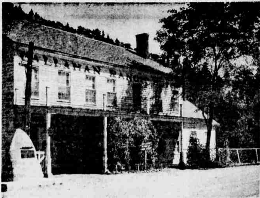
CALLAHAN RANCH HOTEL has stood about like this since gold mining days. It is one of Siskiyou County's historic landmarks, as shown by the monument erected at left. — Photo by Peggy Walsh.
