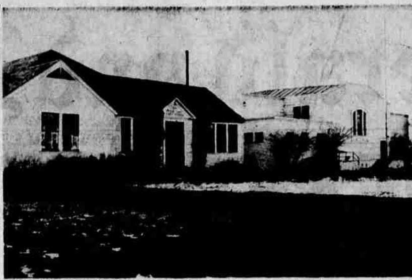
FIRST TULELAKE HIGH SCHOOL, abandoned and windowless, is an eyesore in the center of the town. The school was built in the early day of the town's history on land provided by the U. S. Bureau of Reclamation which provided land for a town-site when Tulelake Basin was opened to Veterans of World War I for homesteading. Veterans received land in other openings as late as 1948. Attempts to settle country by homesteading in earlier years were not successful.
