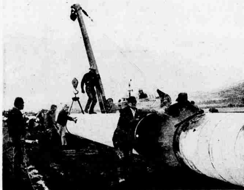
THE SKILL OF PIPELINE MEN is demonstrated here as a lineup crew wrestles a section into position. Most pipeline workers follow jobs around the country, but some unskilled and semi-skilled workers are hired locally. The pay is relatively good but men are separated from their families for long periods and must work under adverse weather conditions.
