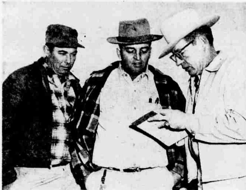
AN INSPECTOR ON THE JOB is a familiar sight up and down the 1,400-mile long Alberta-California Natural Gas Pipeline. Here, inspector W. R. Frisinger checks specifications with two foremen, F. B. VanBenthuyzen and W. D. Scott. The pipeline must meet rigid specifications to perform satisfactorily in all type of climates and conditions.
