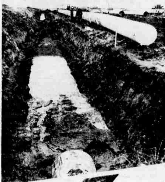
WATER AND MUD in the ditch is one of the biggest problems a pipe laying crew must deal with. Here, Western Pipeline Co. officials inspect the ditch after an early December rainfall. The company keeps large pumps on hand to keep the ditch free of water.
