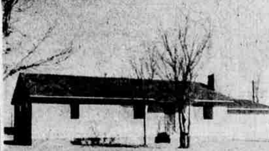
A RESIDENCE for the timber management assistant and his family has also been constructed recently at the Mt. Hebron Ranger Station. This brings to five the number of residences on the station.
