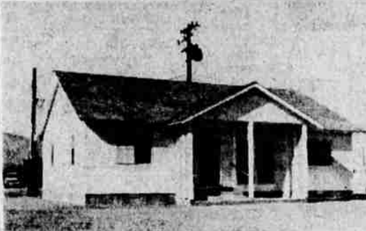
A MODERN five room office has replaced the old office building for the U.S. Forest Service at Mt. Hebron, California. The new building is shown here nearing completion.
