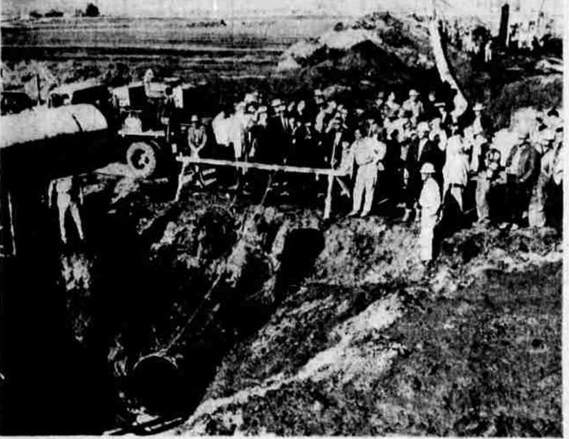
picture shows part of the large crowd which watched the ceremony observing as pipe is lowered to be placed in a casing beneath the road, which marks the border. The line can be seen stretching north toward Bonanza. In the picture at the right, Klamath County Commissioner Frank Ganong presents Senator Arnold with a gift package of Klamath Gem potatoes and wild plum jam. The dignitaries met at a luncheon in Klamath Falls after the ceremony to consider the future of the pipeline. Senator Boivin, Commissioner Ganong and Klamath Falls Mayor Lawrence Slater agreed that the line should provide a substantial boost to the Klamath Basin economy.
