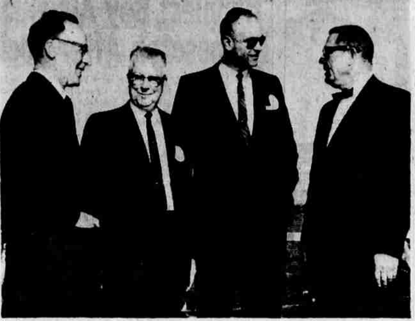
AN HISTORIC EVENT took place Wednesday noon on the Stateline Road east of Malin when the first United States section of the giant Alberta-California Natural Gas Pipeline was dedicated and placed in the ground. The ceremony also marked the crossing of the Oregon-California border. Both state governments were represented along with officials from companies involved in the giant project. In the picture at the left, state senators Harry Boivin of Klamath Falls, left, and Stanley Arnold of Susanville, right, discuss the project with H. W. Haberkorn, second from left, and M. H. (Hap) Chandler of the Pacific Gas and Electric Company. The center
