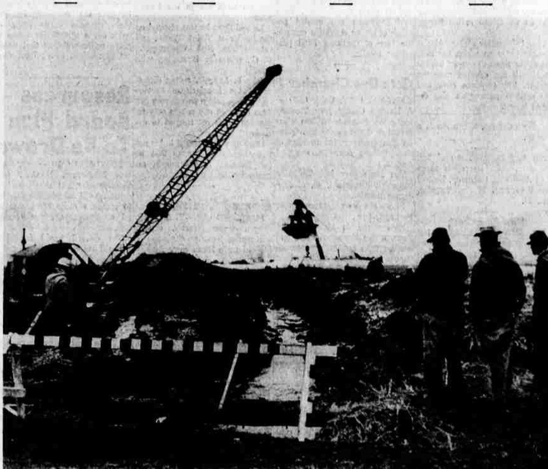
THE FIRST PIPE of the natural gas line being laid in the United States from the Bay Area north to Canada went into the ground shortly before noon today beneath a road lying on the border between Oregon and California. Here, the ditch can be seen stretching away from the state-line road. The pipe is ready to be shoved through a larger culvert beneath the road and then welded to the long piece of pipe stretching into the distance. Officials from both states were present for the pipe laying ceremonies south of Malin. The line will be laid at the rate of 8,000 feet per day and is scheduled for completion in late 1961.
