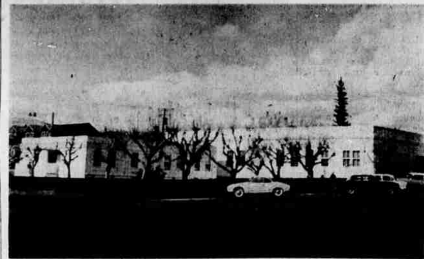
NEW ALL-WOOD office addition (left) at International Paper Company's Weed Branch features interior decorative wall paneling of several wood species. The recently completed structure is connected to the larger original IP office building.
