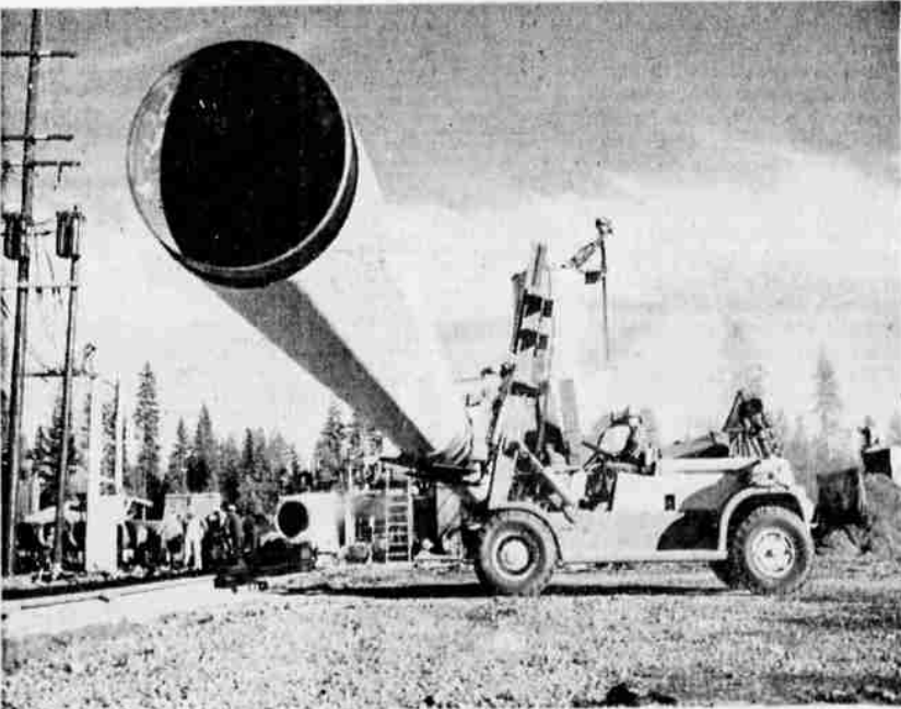
YARD-WIDE PIPE for Pacific Gas and Electric Company's 300-mile long section is being welded into 80-foot sections and treated with a protective "osmotic coating" by H. C. Price Company workmen shown at work at Burney, Calif. The construction team of Western-Nilling and subcontractors are clearing, grading and preparing trench for the first laying-in of pipe for the Pacific Gas Transmission Company's section of the 1,400-mile pipeline at the Sprague River siding. Stanley-Bledsoe and Company are doing the double-jointing and wrapping there.
