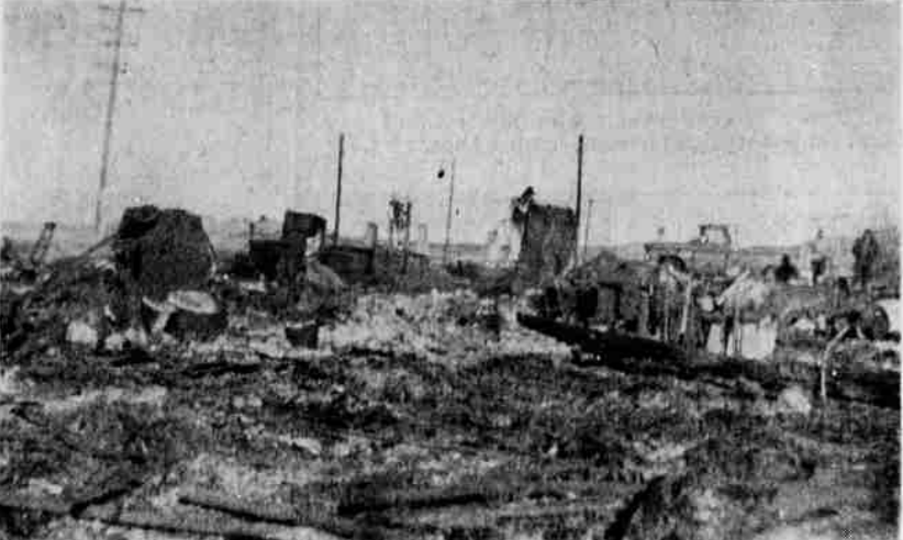
NOTHING IS LEFT of the old Betty Store except the rubble left in the wake of a fire Sunday night. Firemen from several departments and nearly everyone in town tried, but were unable to save the structure.
