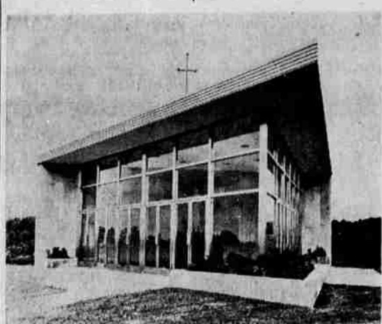
A NEW APPROACH in church architecture features this triangular structure on the campus of Seton Hill College. It is St. Philomena's National Shrine built in the shape of a triangle to symbolize the Trinity.
