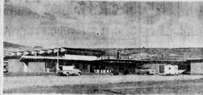
A TRIM, LOW PROFILE distinguishes Falcon Heights School that will open soon. The sawtooth roof in back covers the multipurpose room.
