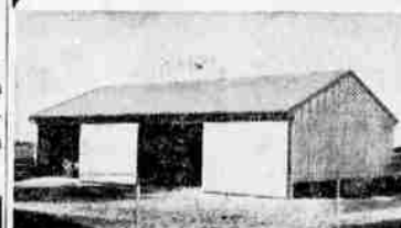
Machinery and Equipment Building
