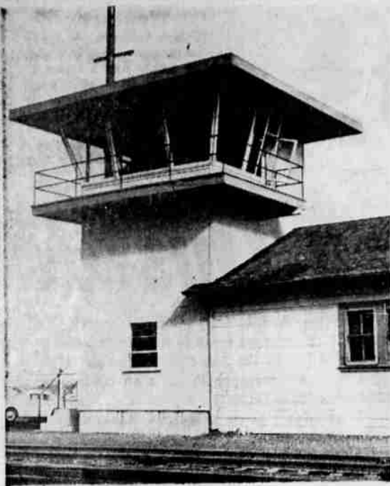
THE CONTROL TOWER at Southern Pacific Company's Klamath District yards here was credited with helping the Shasta Division win the President's Award for safety this year. The division's record was better than that of any other of the company's 11 divisions. From here E. F. Ramsey, general yardmaster, can follow activities on the tracks.
