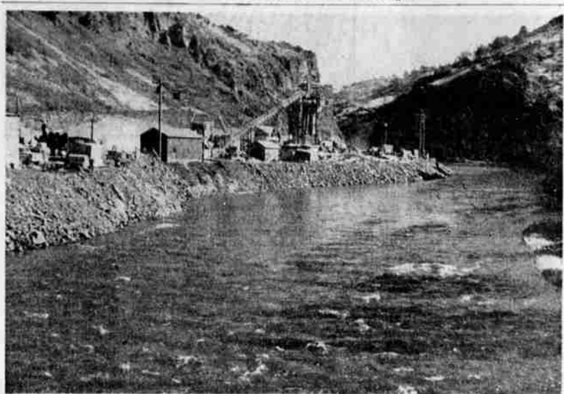
IRON GATE DAM is gradually taking shape in the Klamath River Canyon about 10 miles above Hornbrook. Morrison and Knudsen are constructing the dam at a cost of about $6,600,000 and it is expected that the dam will be on the line by late 1961, producing an estimated 18,000 kilowatts of power. — Photo by J. O. McKinney
