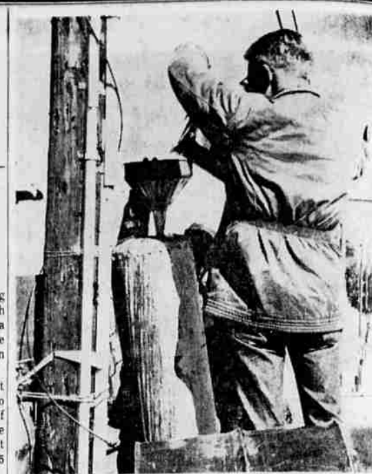
GORDON DARLING, maintenance cable splicer for Pacific Telephone-Northwest in Klamath Falls, pours acetone into old hot water tank used in unusual process to remove water from buried telephone cable.
