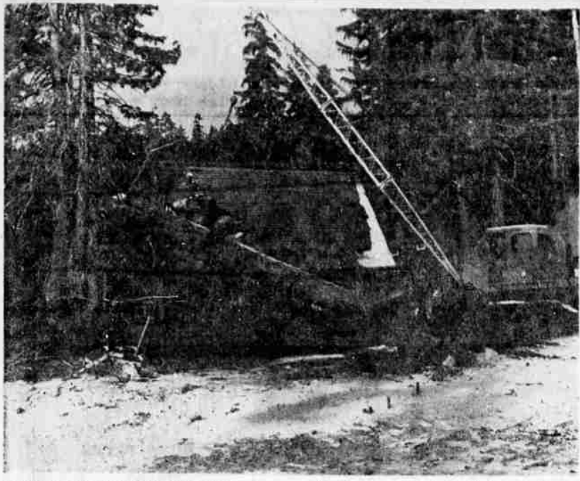
CRATER LAKE HEADQUARTERS took a pounding from a wind storm that roared down the Annie Creek gorge last Sunday. Here workmen are preparing to remove a big hemlock that cracked through the roof of a home — one of three damaged. — Photo by Bruce Black, park naturalist.
