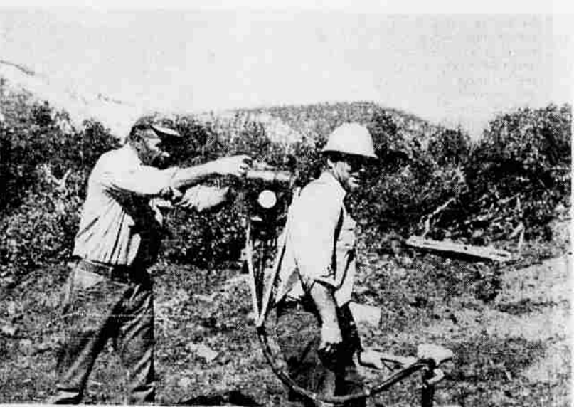
IT'S A TWO MAN JOB to start the soil auger after a change of operators. Here J. C. Bell is about to take his turn at the chore. —Photo by Trickey
