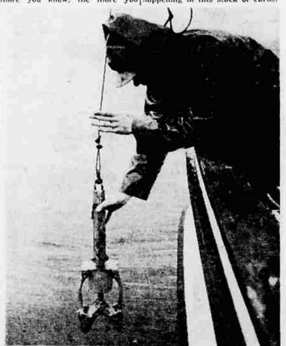
A BOTTOM SNAPPER , device that bites into bottom sediment and brings up samples for analysis of ocean floor, is lowered by oceanography student from converted fishing craft off Yaquina Bay. An 80-foot research vessel to be built this year for the OSC oceanography department will be research source for geologists, biologists, health and fishery people.
