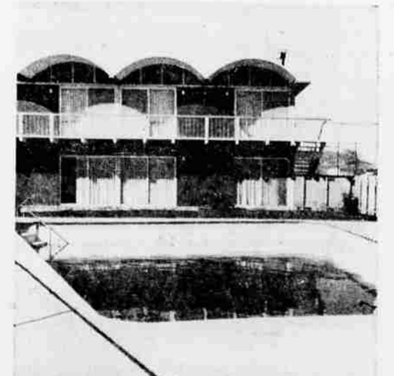
This big, heated swimming pool is available for the exclusive use of Rickfalls residents.
