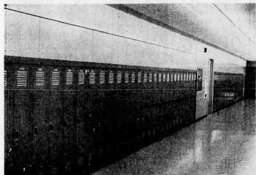
Above, one of the wide, uncluttered, well lighted hallways, with built-in steel lockers.
