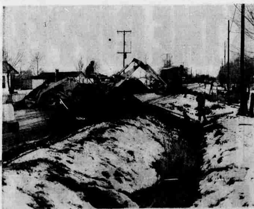
SOUTH SUBURBAN Sanitary District crew lays a sewer line beneath Alturas Drive. This photograph, taken recently, illustrates a scene familiar to suburban residents for more than two years.
