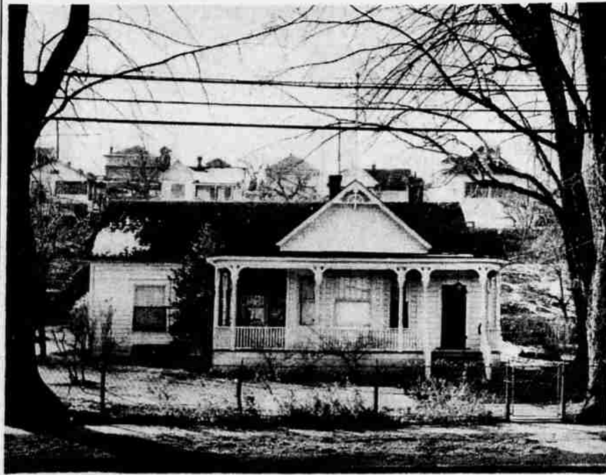
HISTORIC RUFUS MOORE HOME on Riverside Drive in Maple Park is being remodeled to be used as a workshop in connection with the art gallery. The home was built about 50 years ago and is much as it was when Mr. and Mrs. Moore lived there.
