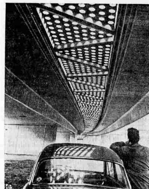
DOUBLE USE —Glossed center stripe of new elevated highway in Dusseldorf, West Germany, provides light for parking below and acts as a divider on surface.
