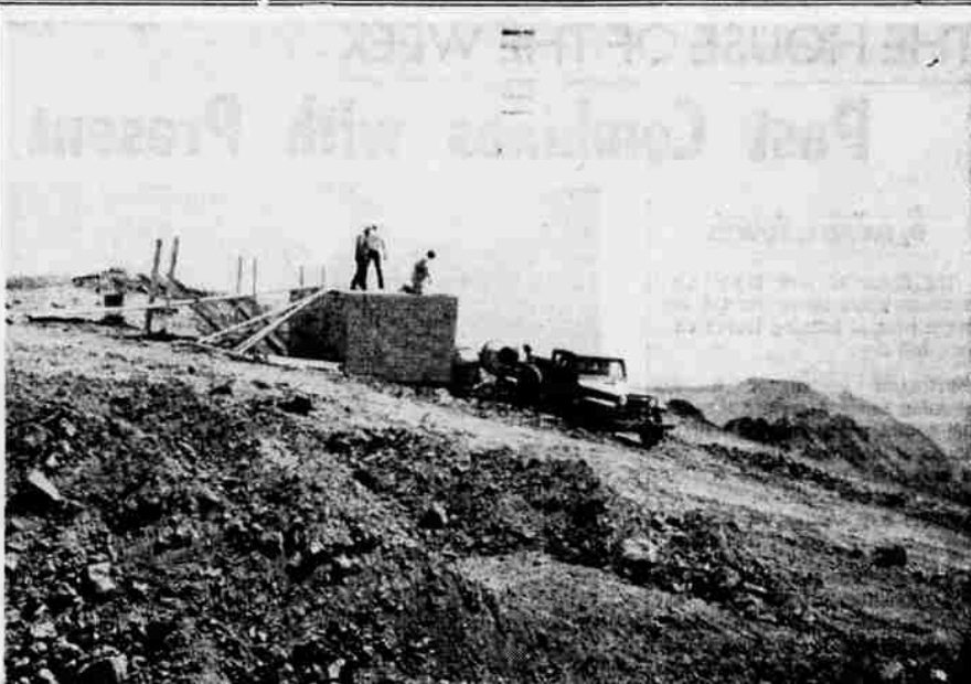
SHOWN HERE ARE BUREAU OF LAND MANAGEMENT MEN constructing two concrete block buildings to house the Wild Horse Rim radio repeater set and a diesel powered generator at the 9,300 foot level on Steens Mountain. The summit of Steens Mountain is the highest point in southeastern Oregon. The Alvord Desert lies 3,000 feet below the station near the foot of the sheer east face of the mountain. Three states, Idaho, Nevada and California, in addition to most of southeast Oregon can be seen from the point. The repeater station has tied together, communication-wise, all five of the BLM Oregon grazing districts within which approximately 20 million acres of land is protected against fire.
