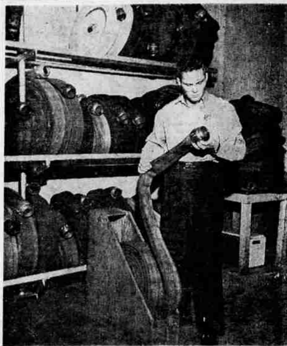
KENNETH FREE, a hoseman, checks the threads on a hose connection before putting it back on the storage rack in the Klamath Falls Fire Department.
