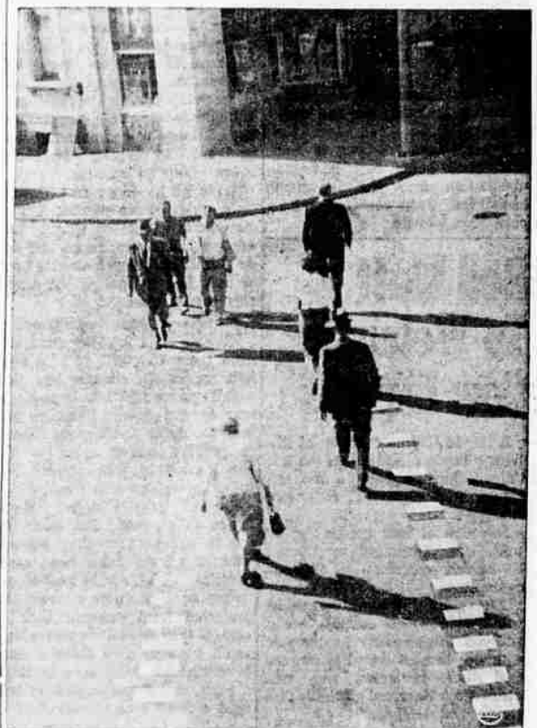
NEW DESIGN SPEEDS FLOW — The inevitable clash of pedestrians meeting head-on in the middle of the street was solved in Madison, Wis., with this new crosswalk design. Two parallel lines of white tile extend from either curb, fading out midway across. A diagonal curb-to-curb line between them forms two "wedges" which, city authorities say, shorten walking time across the street.
