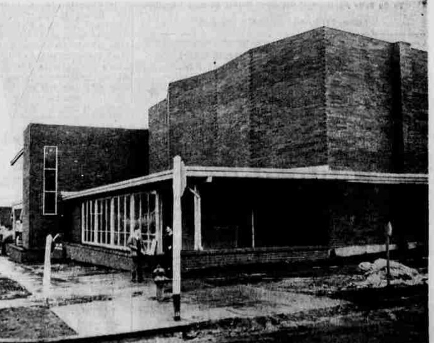
SACRED HEART ACADEMY students and teachers moved into the top floor of the new academy annex last week. The ground floor will be completed soon. Dedication is planned for March. The addition has three classrooms, a science lab and lecture room, a spacious auditorium and other facilities.
